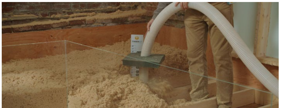
Direct placement method providing better control ►
