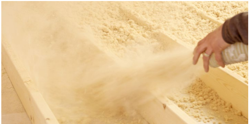
Installation in an open attic ►
